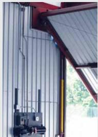
Built for easy access. Cylinders mount inside the slide column. Gives your structure the side clearance and open vistas you want.
